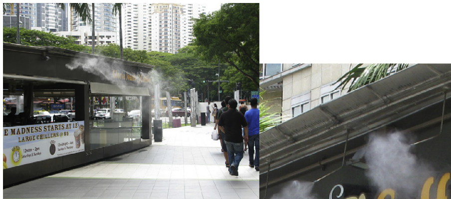
Fig. 3. Misting line system.
